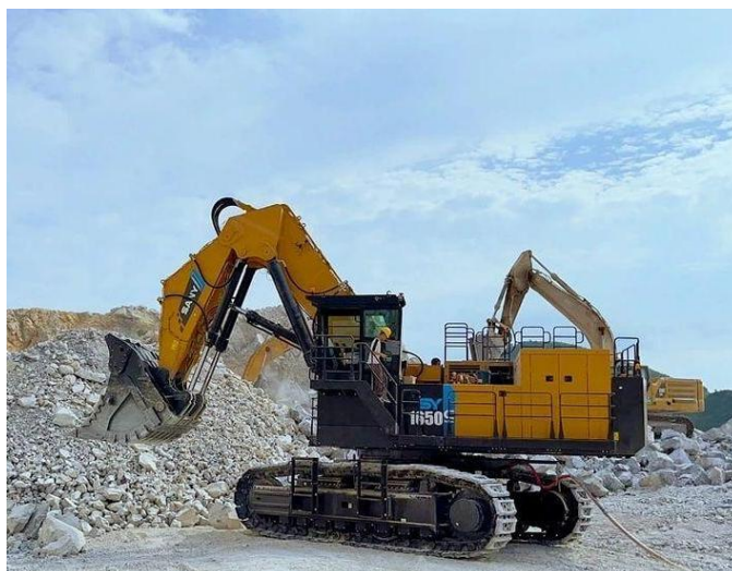
Picture 3.2 – E-10011 excavator
